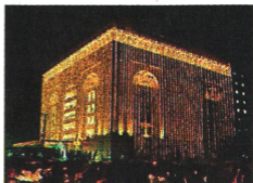
IN ROW: Super Saravana Stores building at Mattuthavani
